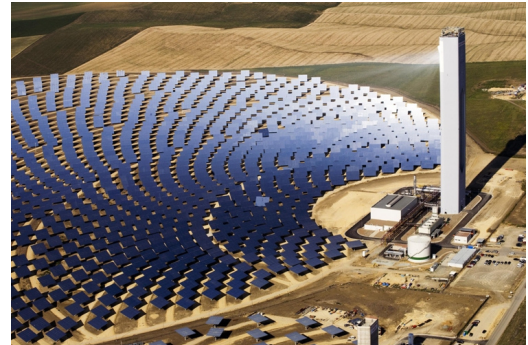
Solar tower power plant PS10 in Spain.
