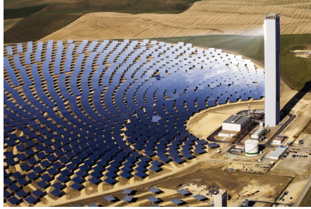
Fig. 1 Solar tower plant PS10, 11 MW in Andalusia, Spain. [Source: flickr]
