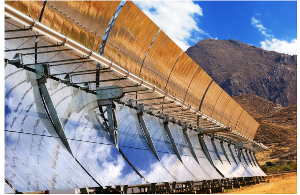
(b) Parabolic-trough solar collector at Plataforma Solar de Almería, Spain [9].
