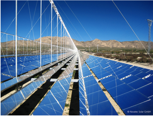
(a) Linear Fresnel collector in 1.4 MW plant PE1 in Murcia, Spain [8].
